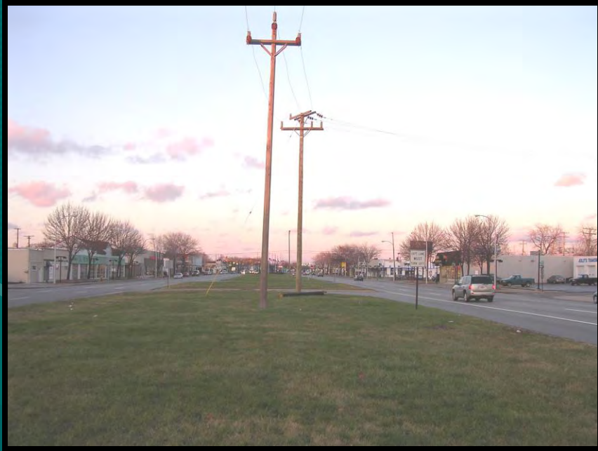
Poor Vertical Containment along Southfield
