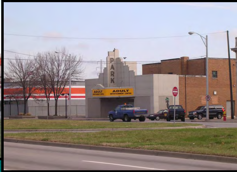
Poor horizontal containment along Southfield
